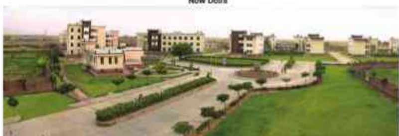
Jagannath University Village Rampura, Tehsil Chakshu, Jaipur (Rajasthan)
